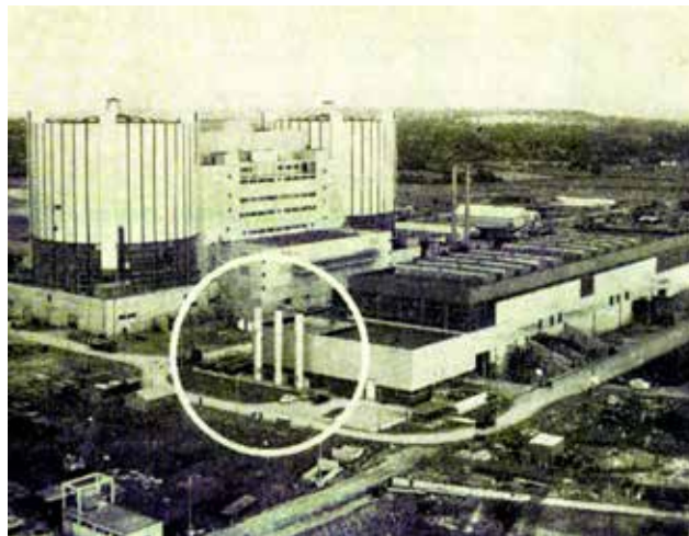
Fig. 20 Gas generator exhaust stacks at atomic power station.
